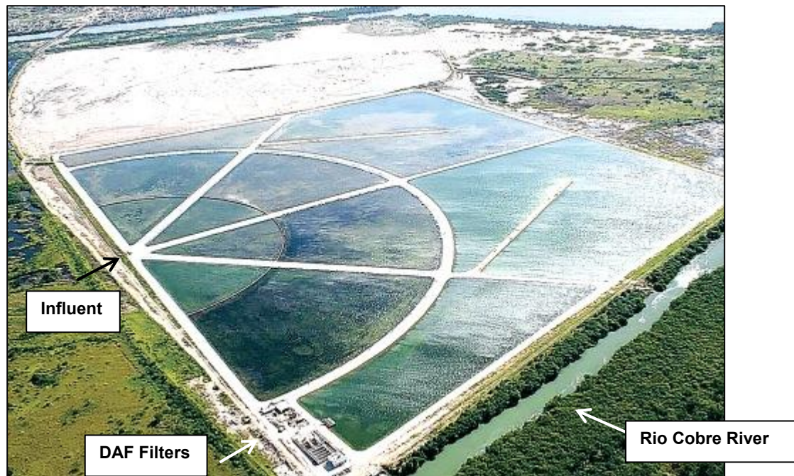
Figure 1.1 Aerial View of Maturation Ponds at Soapberry Water Treatment Plant
